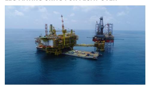
Pioneer 25 years ago for the first floatover installation, Hutchinson has since supplied Leg Mating Units (LMU) and Deck Support Units (DSU) for more than 40 successful installations around the world.
